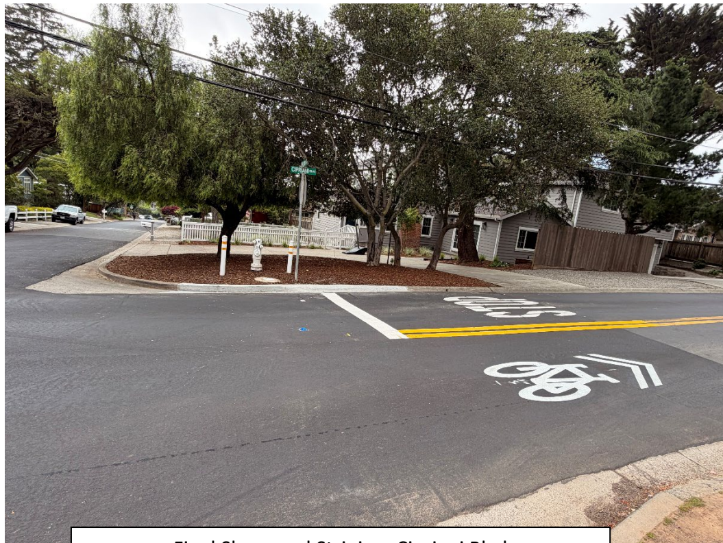
Final Slurry and Striping- Cipriani Blvd
