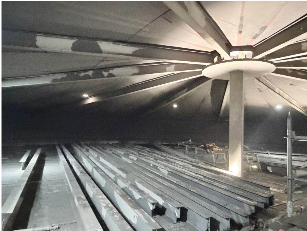
Exbourne (W) – New rafters sand blasted prior to coating.
