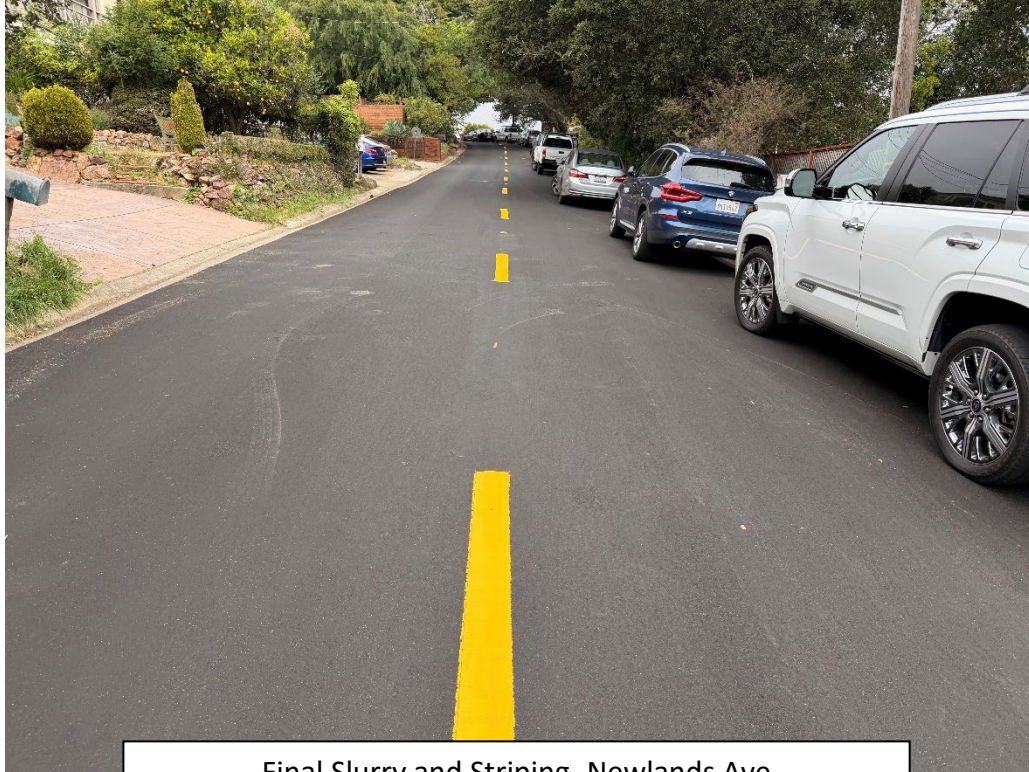
Final Slurry and Striping- Newlands Ave
