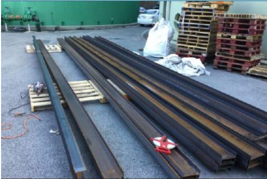
Exbourne (W) – New rafters to be installed.
