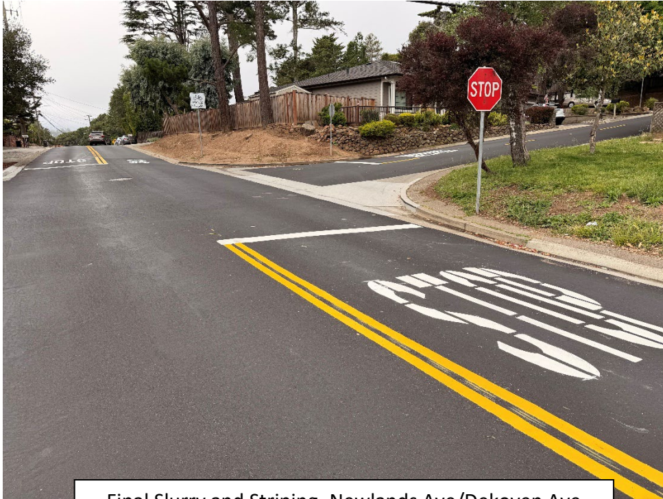
Final Slurry and Striping- Newlands Ave/Dekoven Ave
