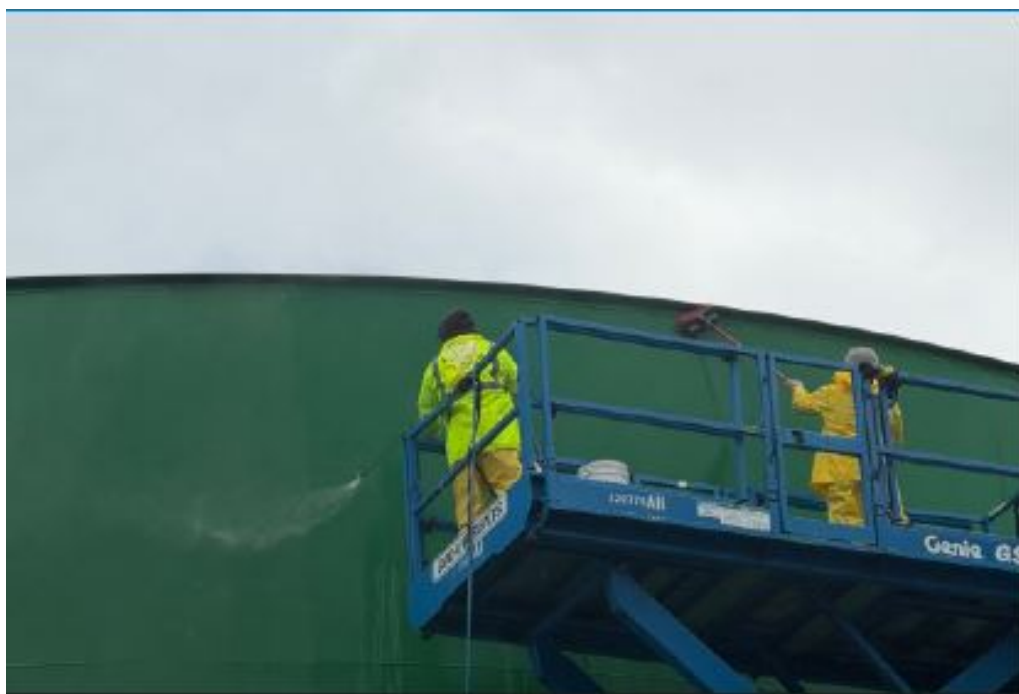
Exbourne (W) – Pressure washing & cleaning the exterior tank shell.
